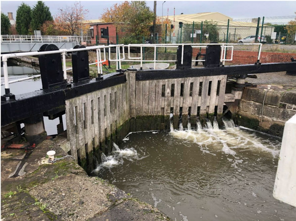
Figure 3 - Downstream face of the top lock gates to be modified at Keadby Lock (image Arcadis 2022)
